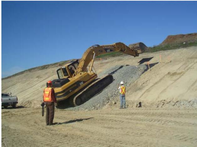
**Test pad under full equipment load.**
