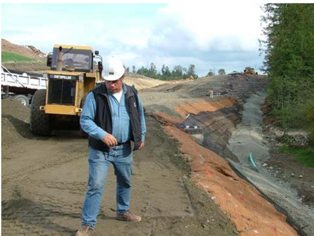
**Geogrid Reinforced Berm under construction.**
