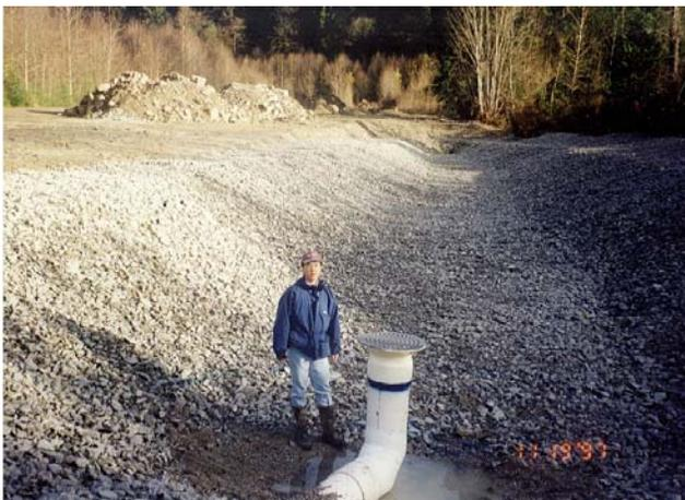
**Rip Rap armoured Sedimentation Pond as Engineered by SHA at Inter River Park.**
