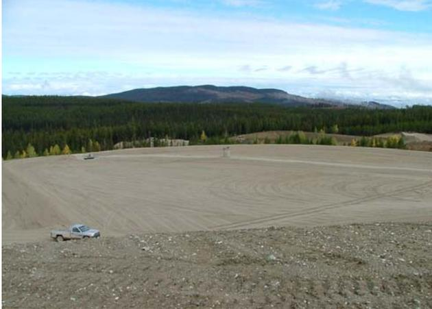
To provide secure leachate containment the landfill has been constructed with a double liner system using 1,000 mm of local glacial till, overlain by a 60 mil textured HDPE liner. Leachate is conveyed to a large double lined leachate storage and treatment lagoon.
